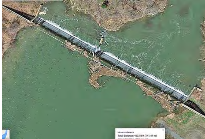
Goose Creek Dam – water flowing
